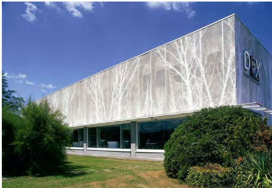
7. SCREEN, PERFORATED METAL - Pic Perf, Locker Group SCRP
