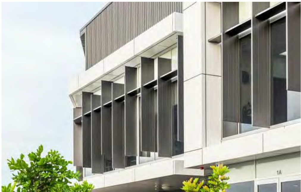
10. SUNSHADE, HORIZONTAL - Aluminium Blades LOUVRECLAD SUNH
