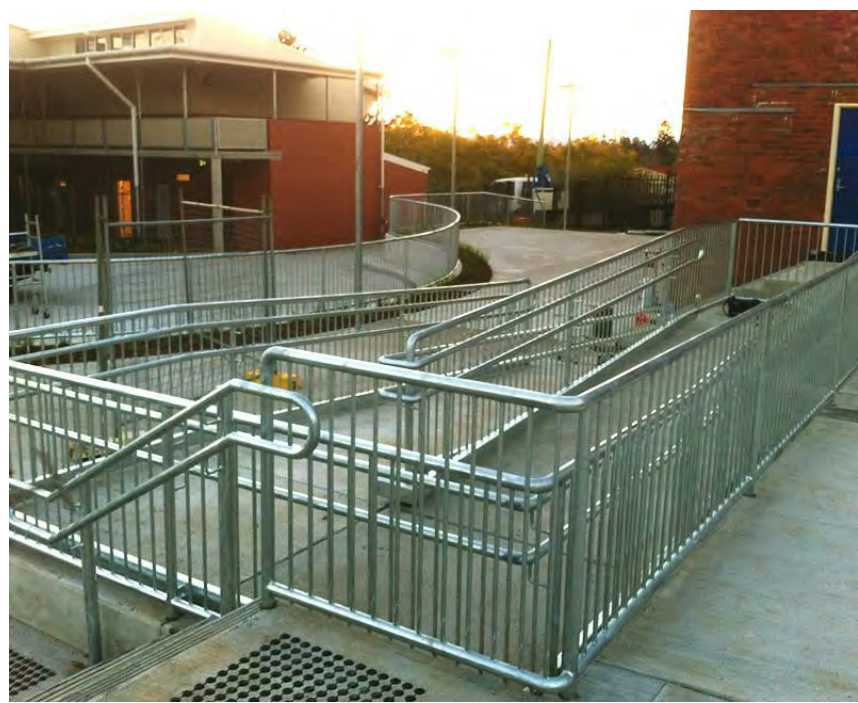
5. BALUSTRADE - Galvanised steel balustrade BAL
